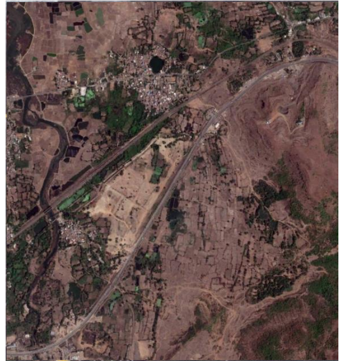
The six-lane road project began in its initial stage, establishing a connection between Pushpak Nagar, JNPT port, & CBD Belapur highway.
